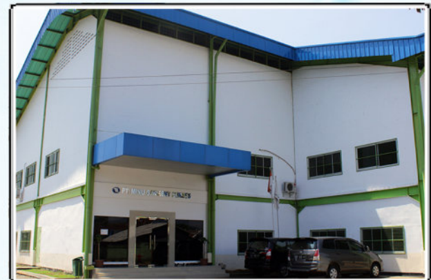
DRY ROOM GARMENT ROOM, FOR CONTROL OF WATER CONTENT BELOW 15 G/KG
